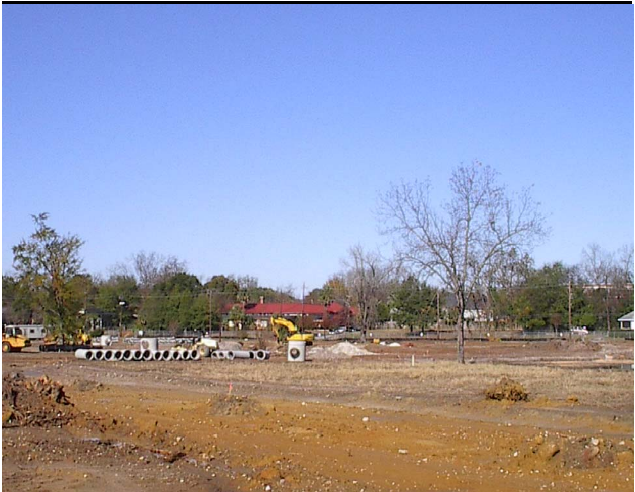
11-29-05 view looking northerly across the work area from Ivy Avenue
