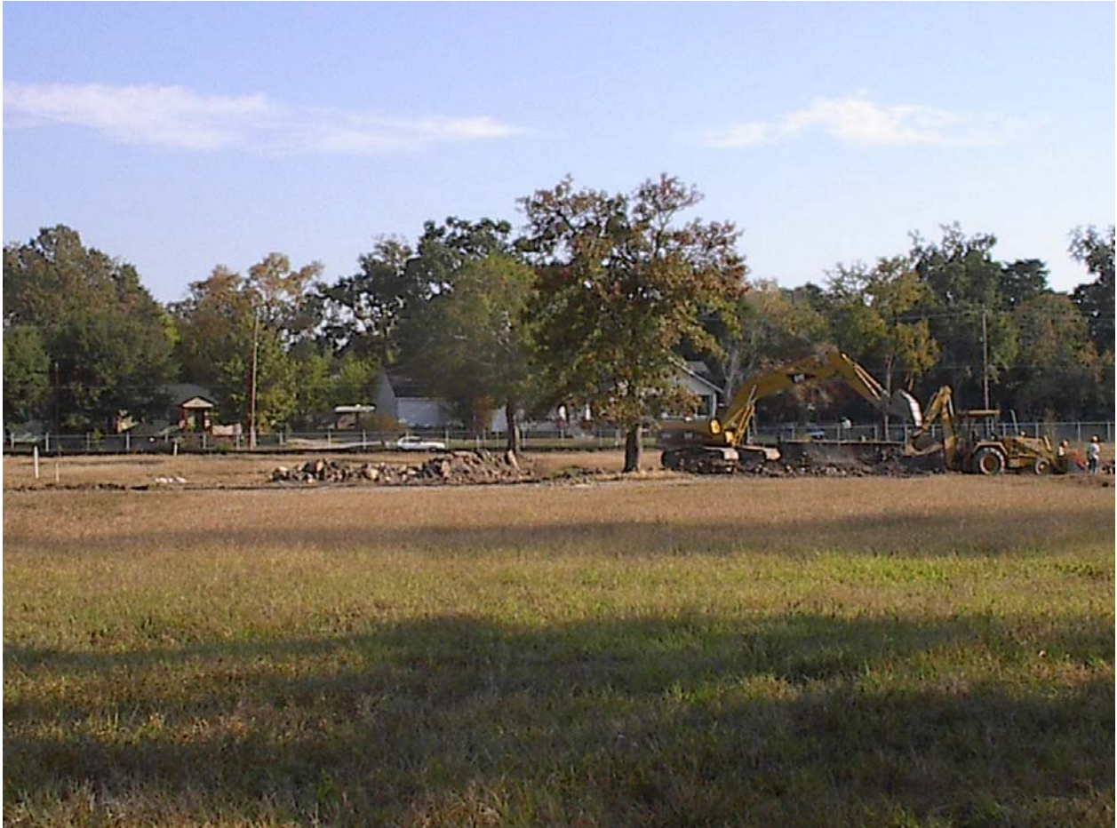
11-02-05 view looking south to north from Ivy Avenue
